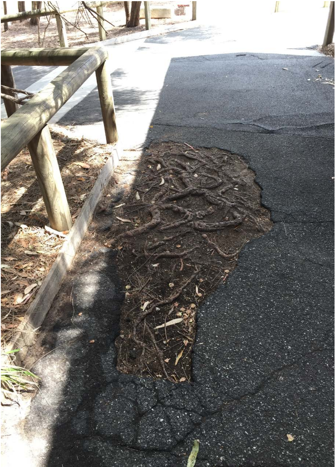
FIGURE 13: TREE 8, EXPOSED ROOTS AND BROKEN PATHWAY SURFACE.
